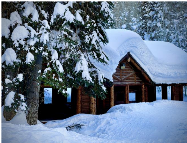
Spruces Campground Pavilion – February 2023
