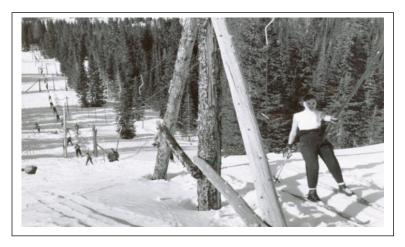
In 1955, Doyle purchased the first two-person chairlift in the Intermountain West and installed it himself. Boring 9-foot-deep holes into the solid granite with a single jack and a sledgehammer for the lift footings took Doyle all summer and resulted in a 50-pound weight loss! It was a smashing success and shortly after, a second double chair, The Mary Chair, was added where today's Crest Express is now.
